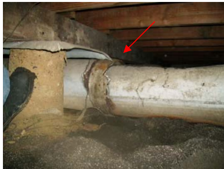
15 drawing air from crawl space
