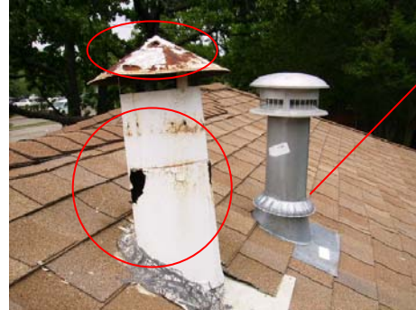
2 holes through old furnace flue
